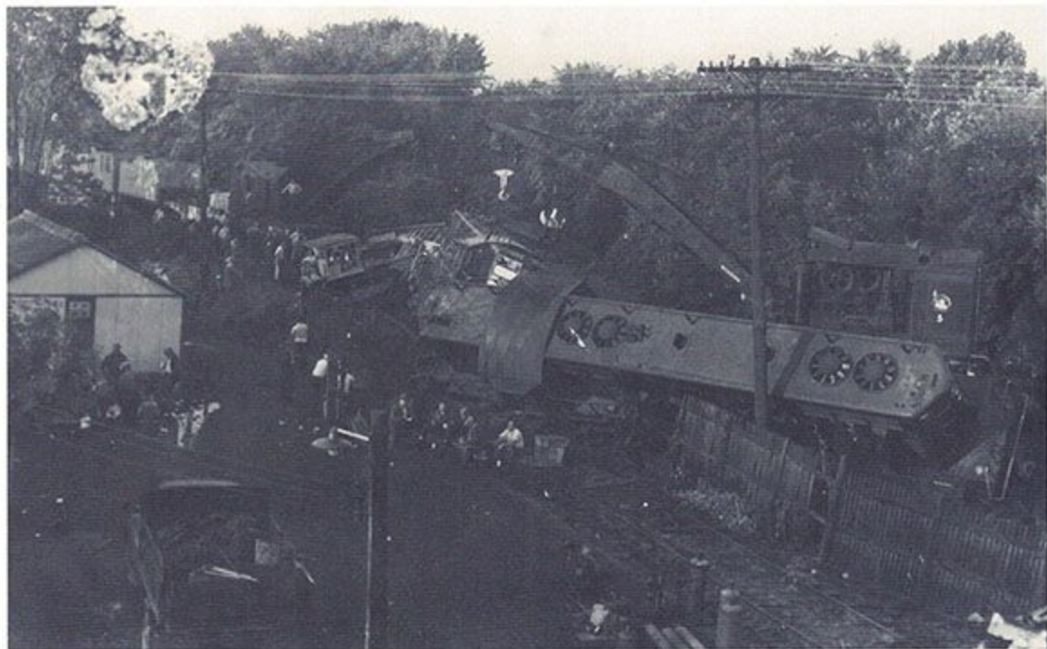
August 1956, Train Wreck on Lower Seventh Street caused $40,000 dollars in damage.
